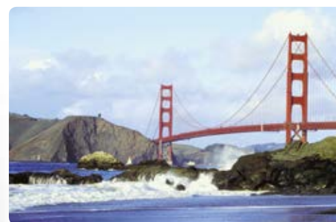
Golden Gate Bridge
